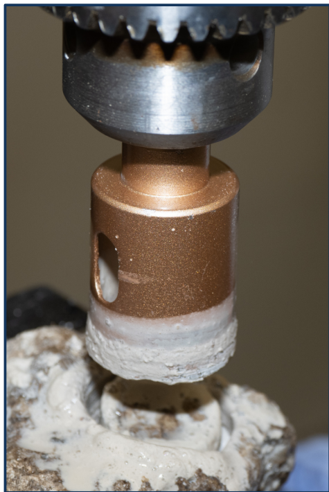
Fig. 3: Coring in process.
